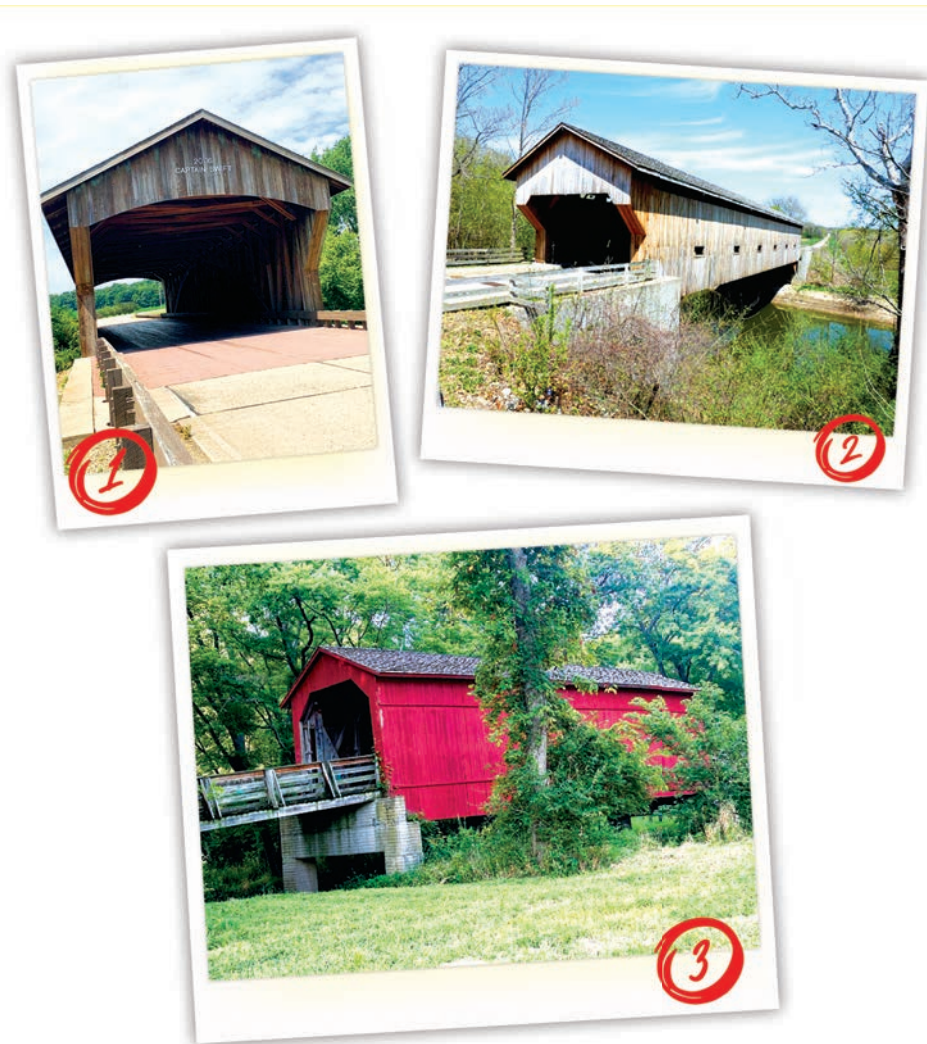
1. Two-way vehicle traffic can pass under the Captain Swift Covered Bridge near Princeton. Another covered bridge near Princeton, the Red Covered Bridge, is closed to traffic after a semi-truck heavily damaged the bridge. PHOTO BY MARY BOHLEN 2. The Cumberland County Bridge near Greenup is an official site on the Historic National Road and spans the Embarras River. PHOTO BY BRENT BOHLEN 3. The Sugar Creek Bridge near Glenarm is a popular stop for travelers on nearby historic Route 66. PHOTO BY BRENT BOHLEN
