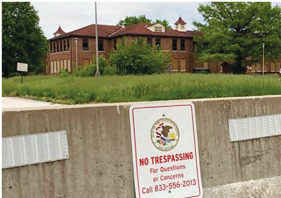
The Jacksonville Developmental Center, located in the center of Community Park, has been closed for 12 years. The 60-acre campus has been the site of at least five suspicious fires within the past five years and police frequently find individuals trespassing on the property, which has no lights, cameras or security system.
