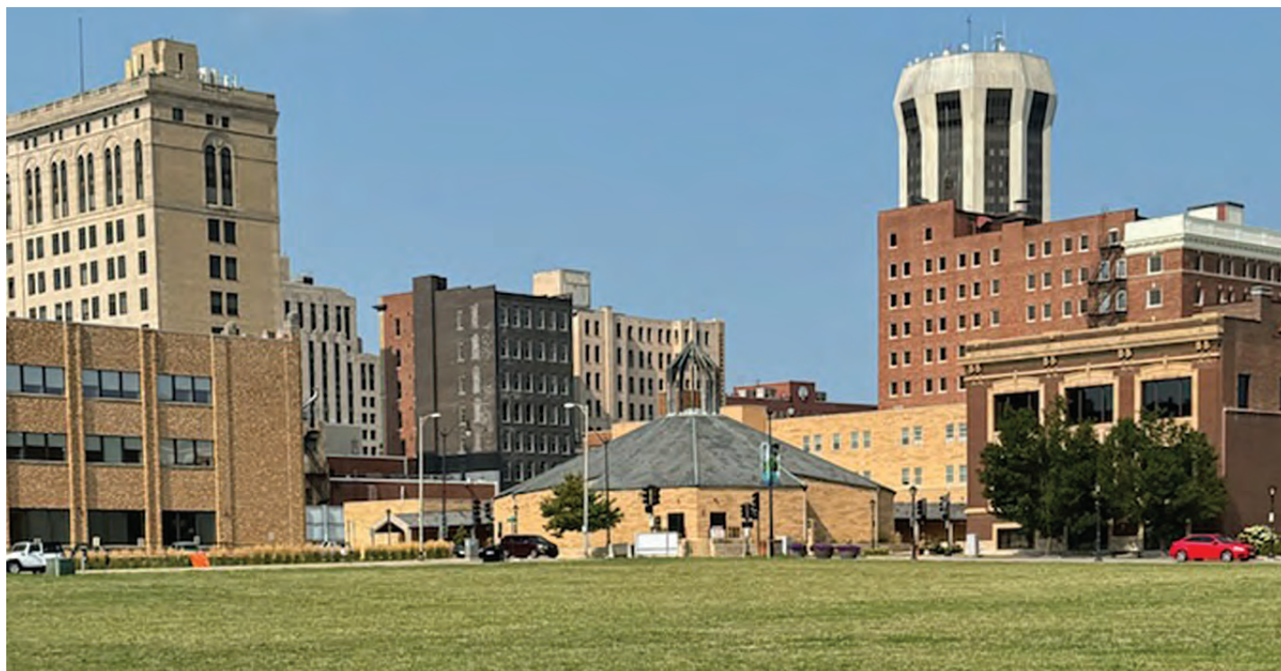
The current state budget appropriated $4 million for "design, construction, improvements and other capital expenditures for the development of the Governor's Mansion block." Mayor Misty Buscher says she plans to make it into a park. PHOTO BY KAREN WITTER
